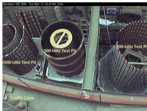
Figure 14.10: 200 MHz test pit (2.5 m diameter and 5 m deep) under construction at Cornell. The other pits are for testing existing cavities.
