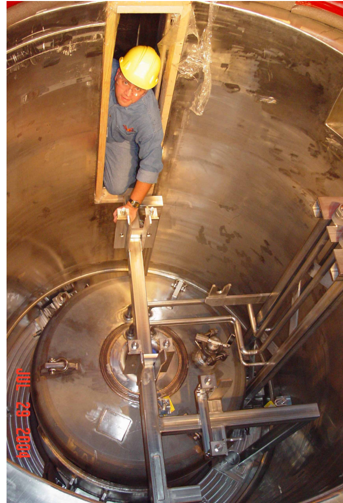
Storage Tank in Collection Basin
