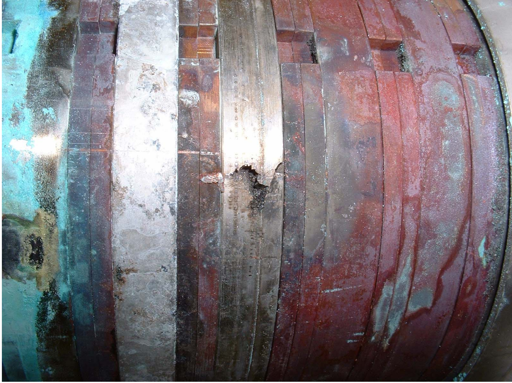
Exit Damage (Jim Morgan)
