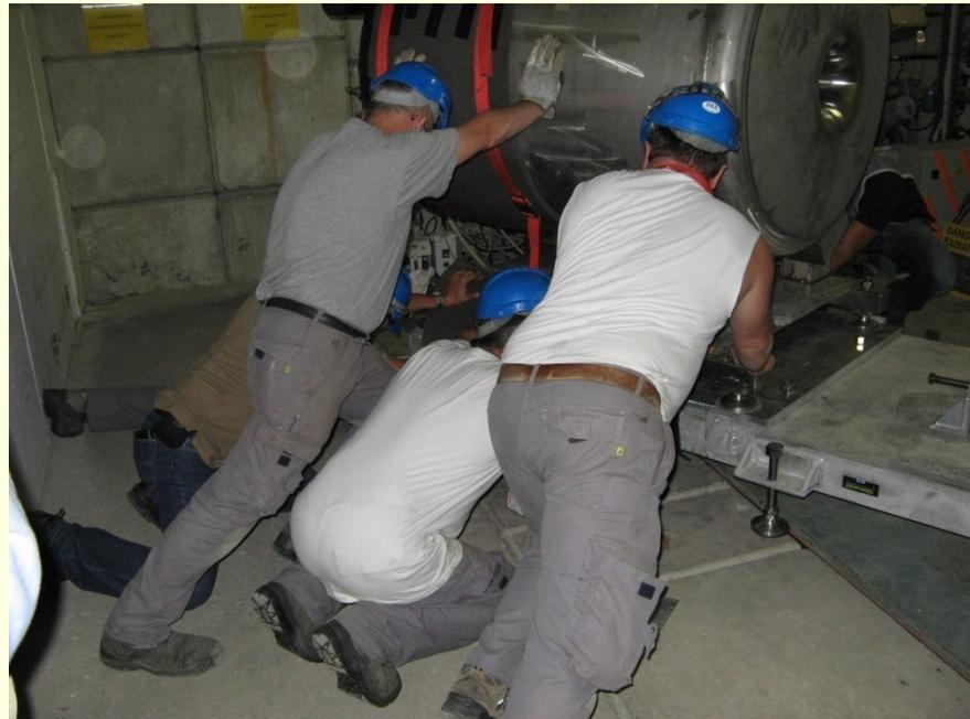
*... down the TT2 tunnel (6% slope, 6T object)*
