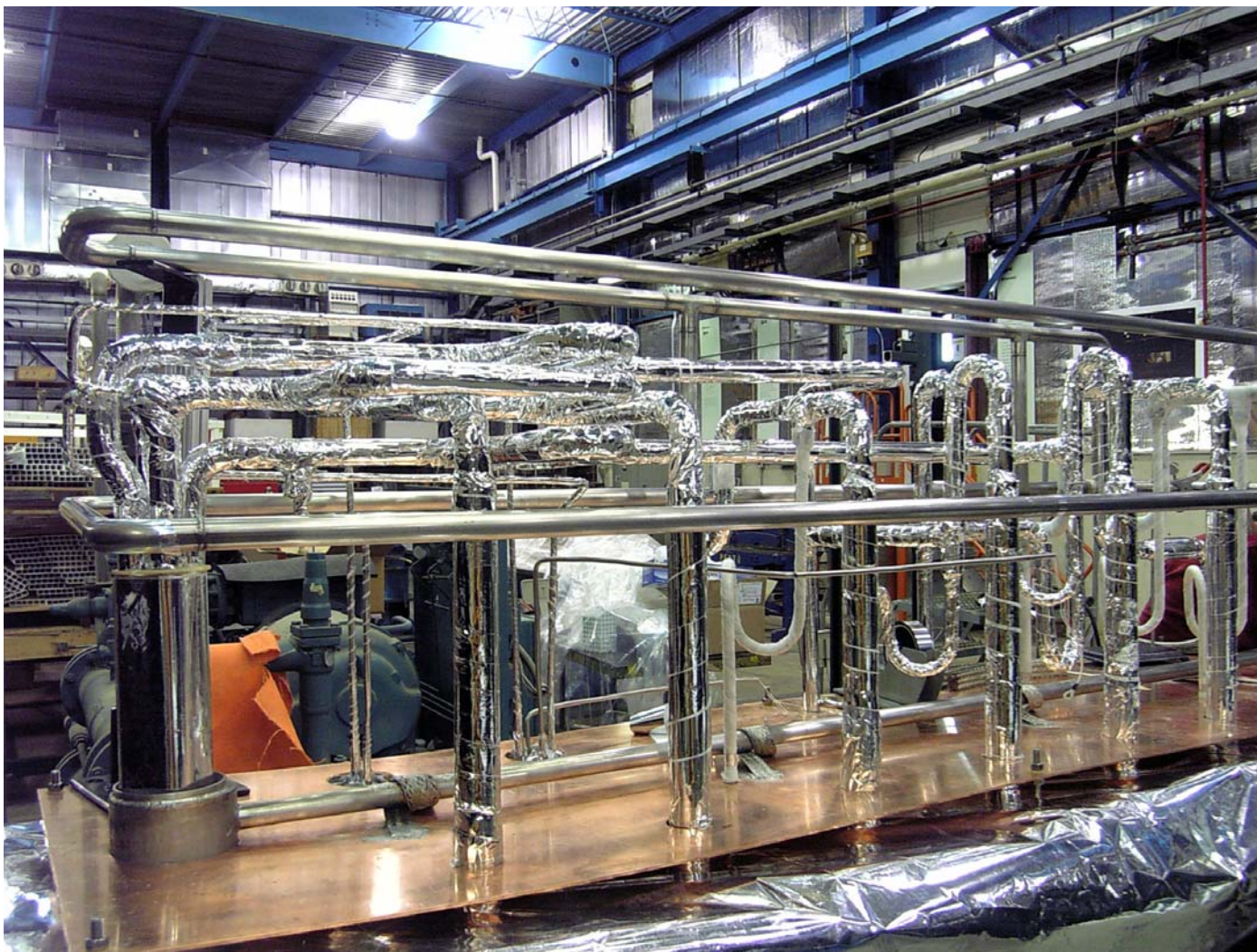
Valve Box Piping
