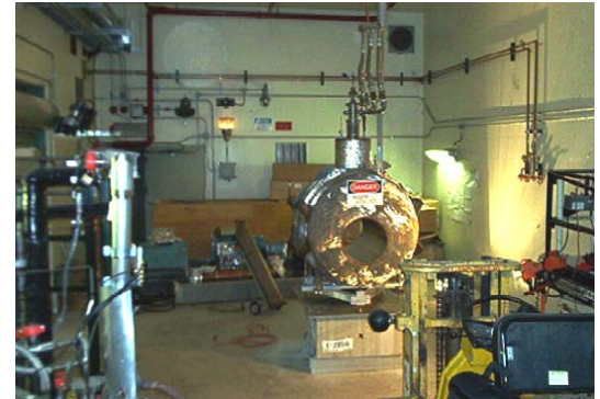
Preparing for RF Testing in MTA
