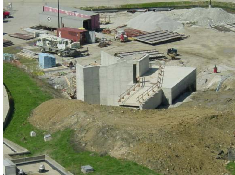
Stage 2 construction area
