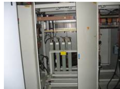
Passive filter capacitors
