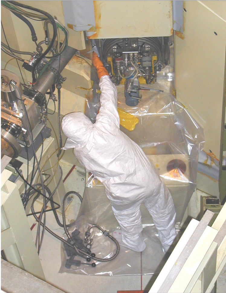
Operation of the remotely controlled shielded flask
