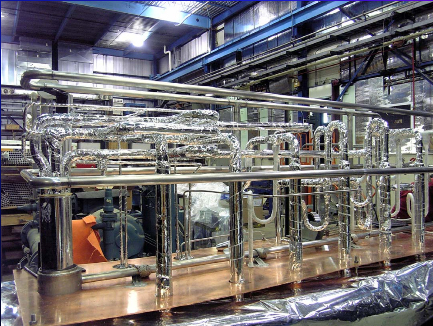
Valve Box Piping
