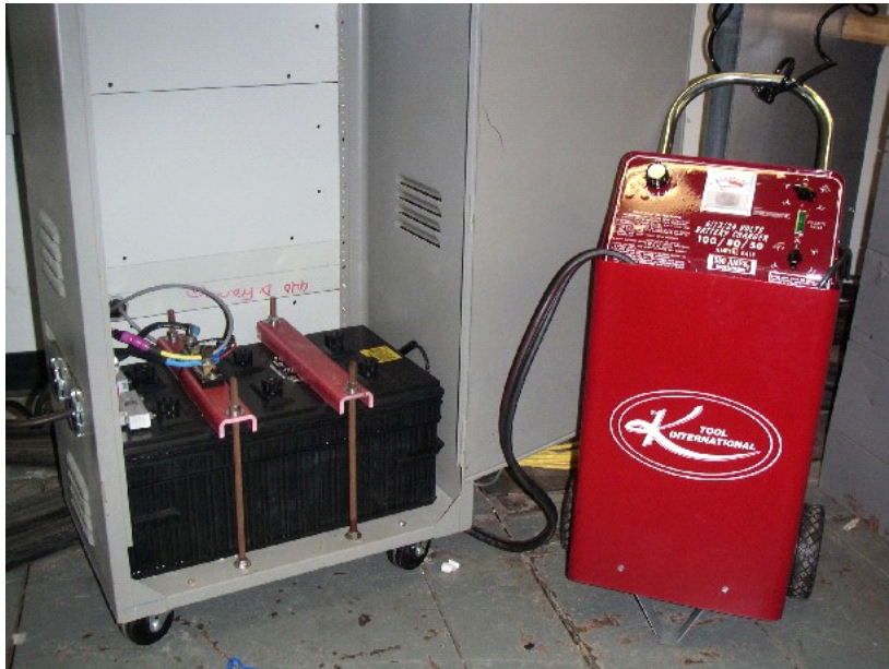
Battery and charger (12 V, 1400 A)
