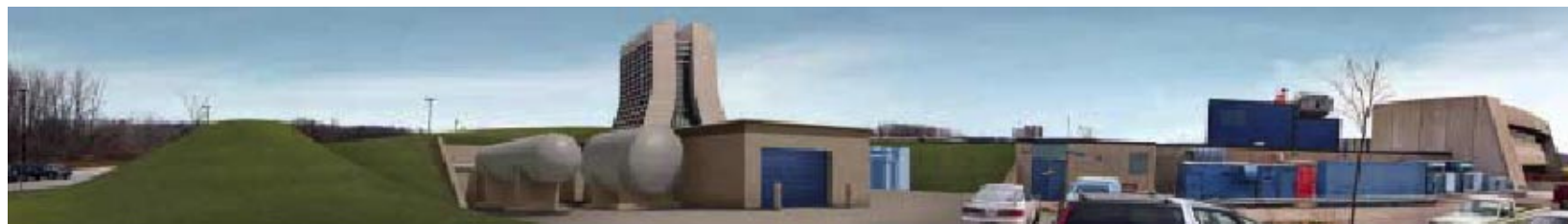
What it will look like when completed
